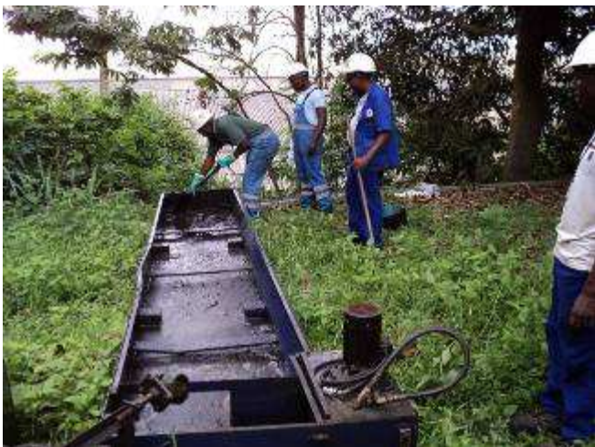
Figure 21: water tank cleaning.
