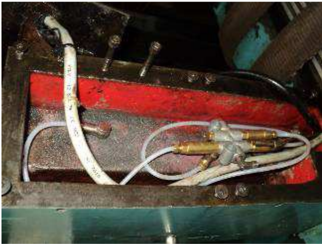
Figure 33: The new Oelverteiler with 2 Dossier units. 2 pieces of type 16 lubricating points, and even a type 10 it.
