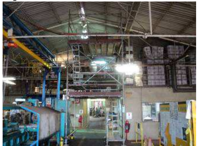
Picture 35a. Located next to the White CNC lathe, a framework was due to a small hole in the roof, installed. As one would build a hotel. This has to do with the fact that here in the camp, the company Chevron, USA, has a strong safety follows thought.
