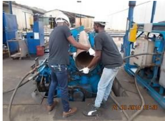
Picture 58) screwed an important machine that pipe threads.
