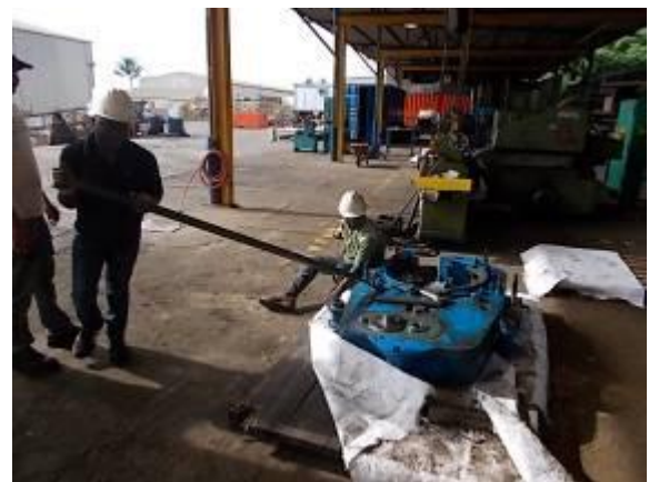
Figure 64) with large extensions had to be opened some of the screws.
