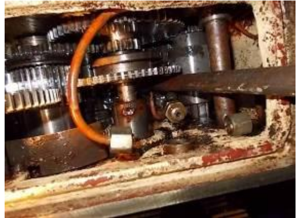
Figure 40) The transmission had a lot of mud and dirt down there. It is impossible to do so to clean without dismantling once each.
