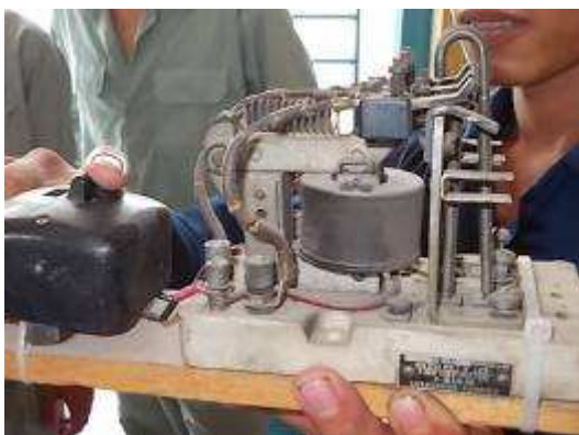
Photo 18: Nice, as here, the function of a contactor is clearly visible.
