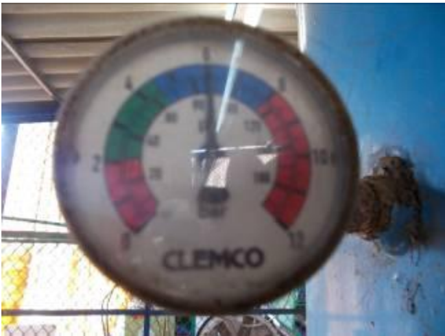
P64: Before starting a test system, if the system pressure corresponds to the pressure.
