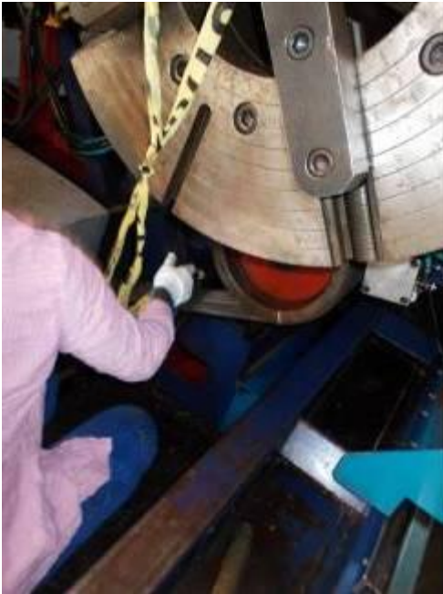
P17: detach the headstock is very difficult. These M24 bolts grade 12.9 must be tightened and loosened on one meter by 94 kg. That takes a lot of force.
